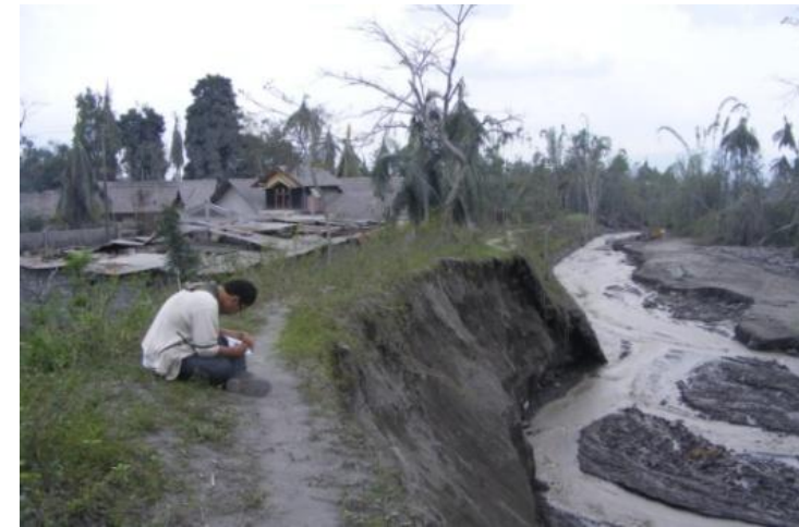
Broken dike caused by lahars in Putih River at Krapyak Village (left & middle), and Karanggowang Village (right).
