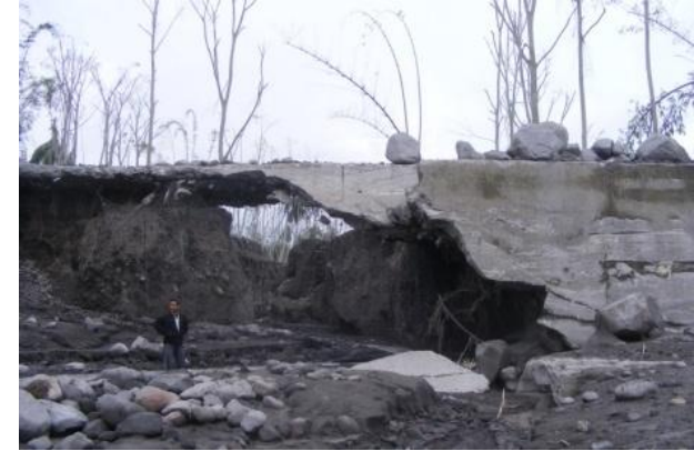
Broken dam due to flowing lahar at Putih River in Sirahan Village (left), Krapyak Village (middle), and Ngepos Village (right).
