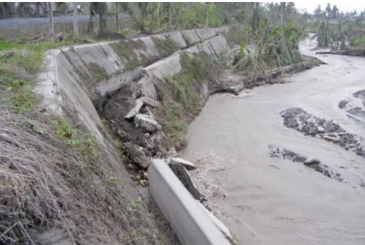
Broken dike caused by lahars in Putih River at Krapyak Village (left & middle), and Karanggowang Village (right).
