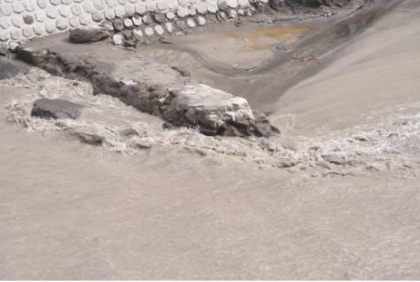
Broken dam due to flowing lahar at Putih River in Sirahan Village (left), Krapyak Village (middle), and Ngepos Village (right).
