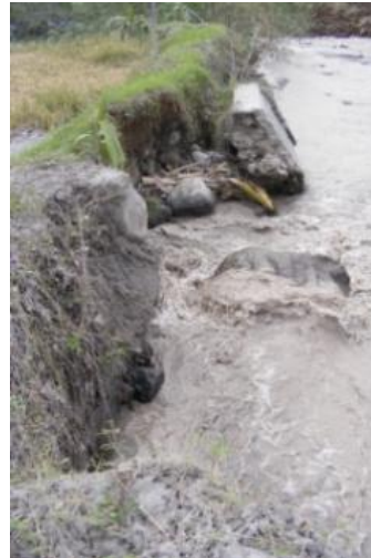
Broken dike caused by lahars in Putih River at Krapyak Village (left & middle), and Karanggowang Village (right).
