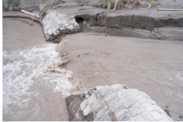
Broken dam due to flowing lahar at Putih River in Sirahan Village (left), Krapyak Village (middle), and Ngepos Village (right).
