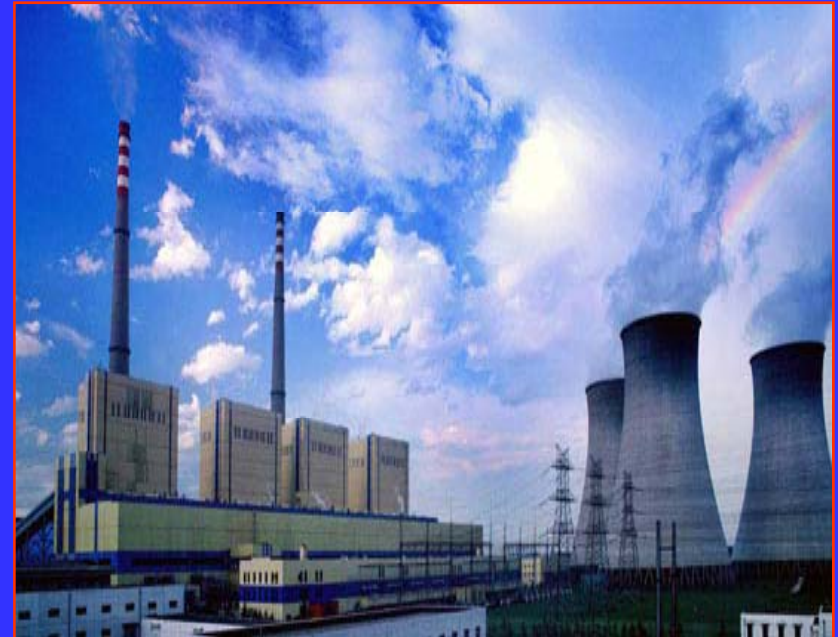
Gaobeidian power plant in Beijing
