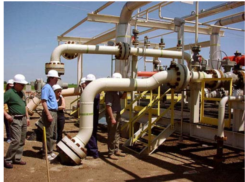
This is where CO 2 arrives after a 320 km pipeline transport from the coal gasification at Beulah in North Dakota, USA
